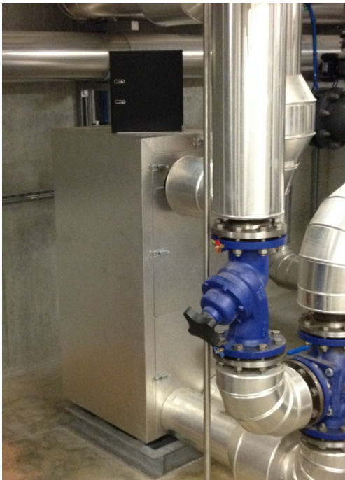
Figur 96 Havvandsveksler, 477 kW
