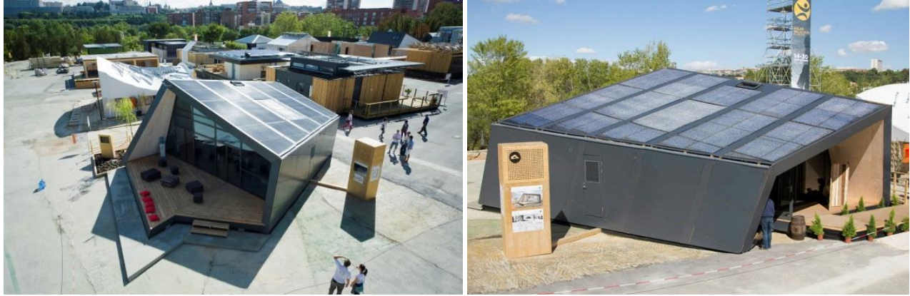
Figure 2. Outside views of the house, seen from North-West and South-West
