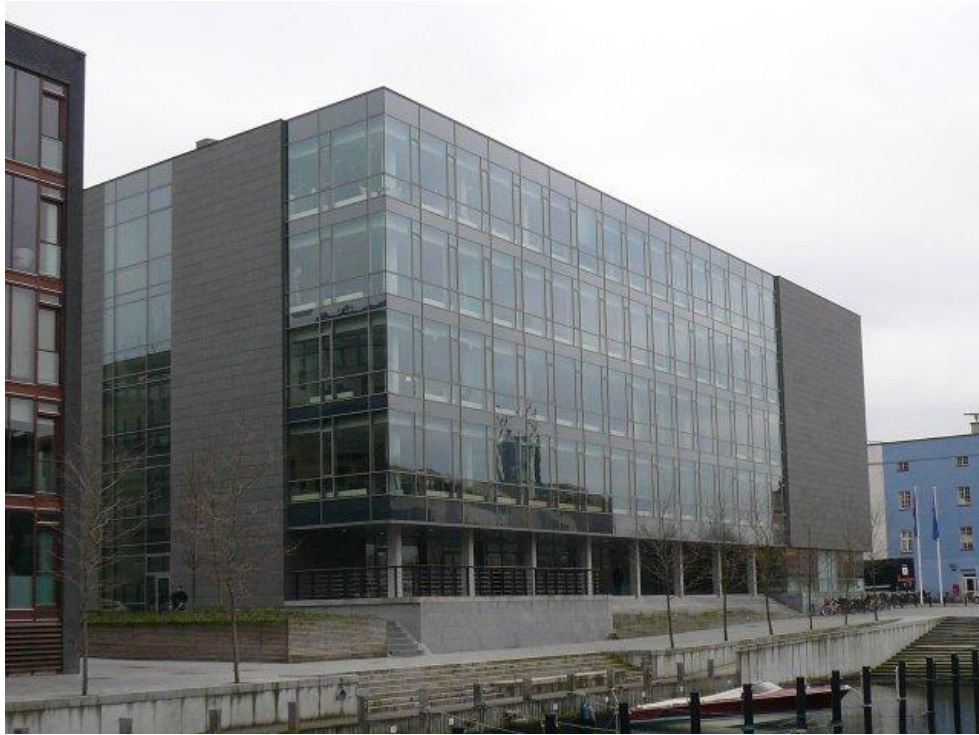
Figure 2.5. The North West façade. Orientation: 35^\circ from North towards West
