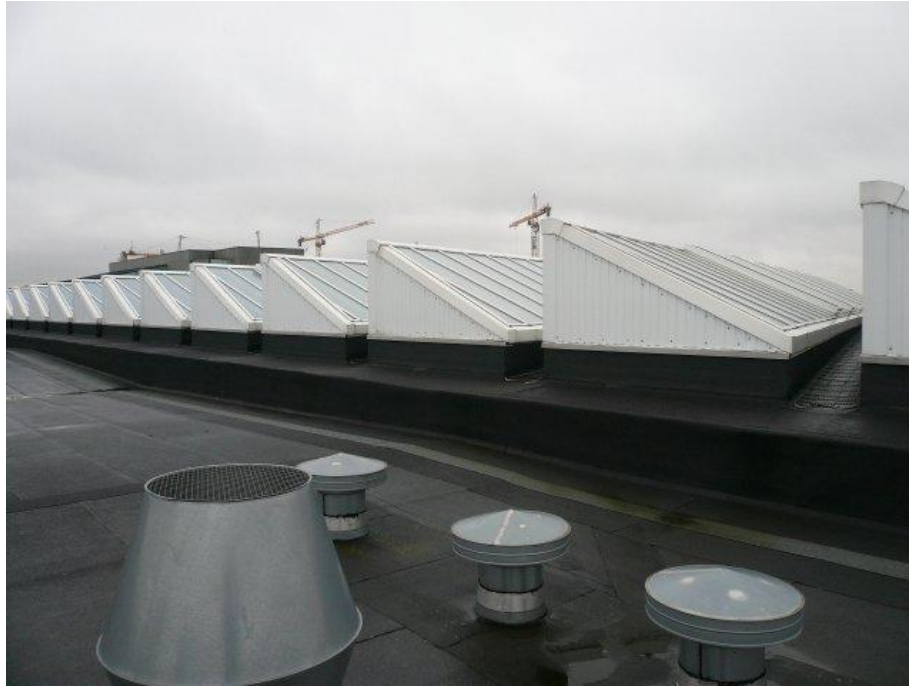
Figure 2.9. The roof of the atrium seen from outside.
