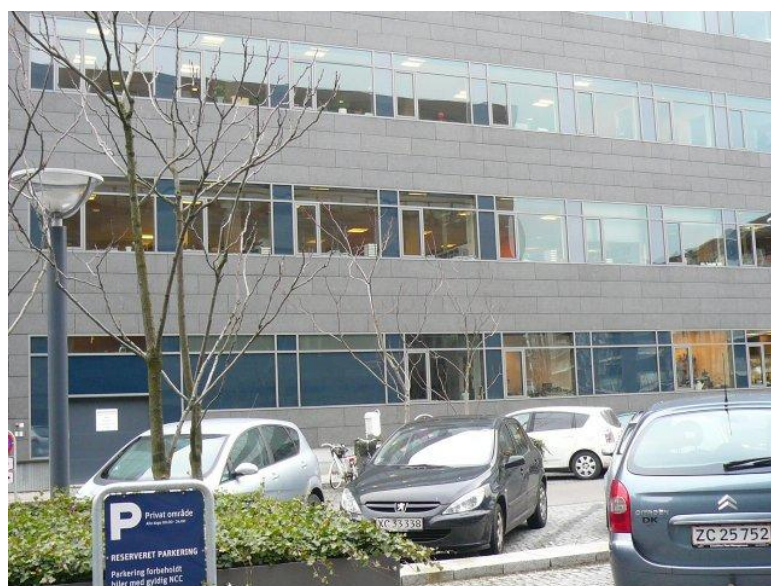
Figure 2.10. Opaque glazing in the façade.
