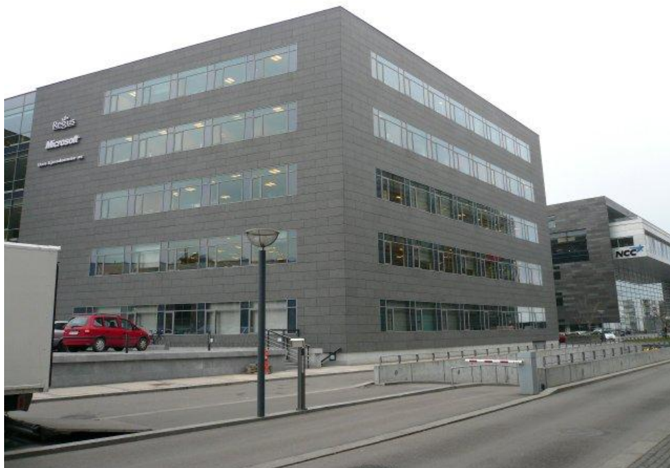
Figure 2.3. The South façade. Orientation: 15^\circ from South towards East.
