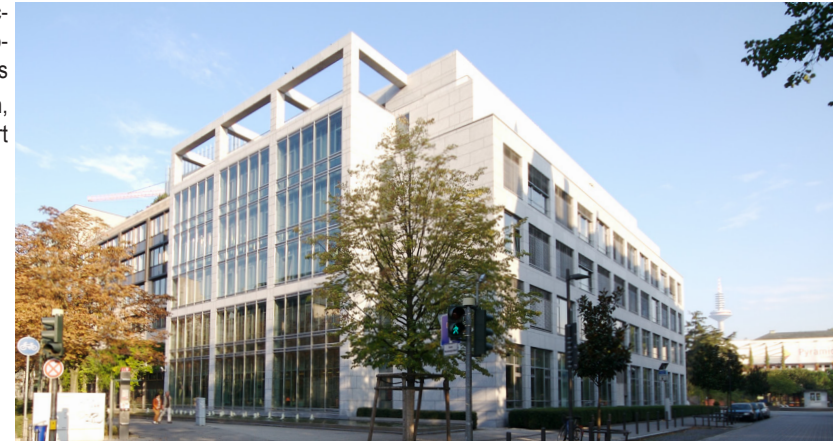
Office focused on electricity efficient equipment and appliances KfW Banken, Frankfurt
