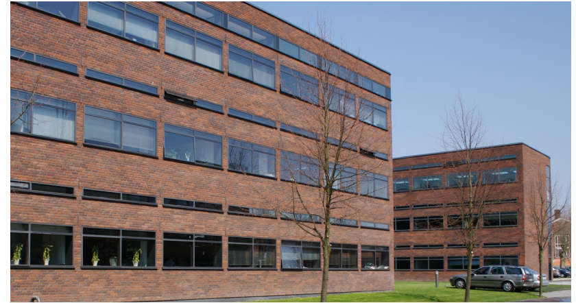
Office building with large thermal mass Pihl & Søn, Lyngby
