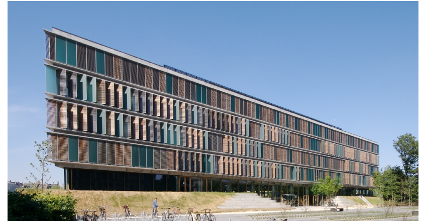
Automatic solar-shading for daylight and indoor climate control CBS, Frederiksberg
