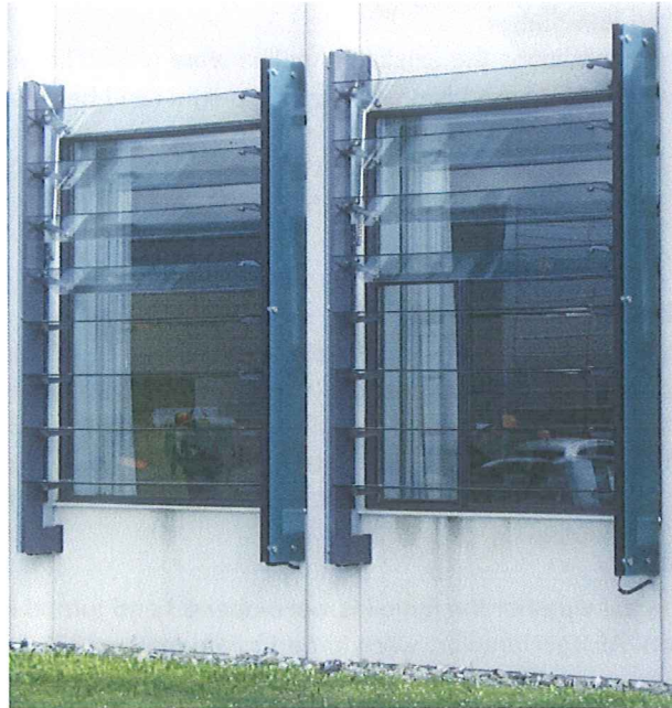
Figure 7. Close-up of glass lamellas in test area. The top four lamellas are made of Antelio Silver glass 10 mm thickness.
