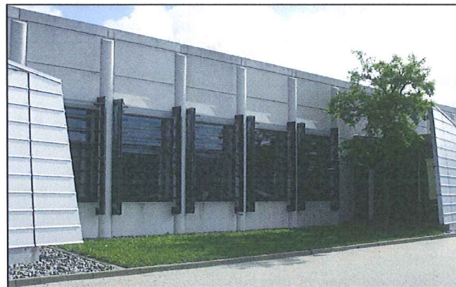
Figure 2. Façade of test area.
