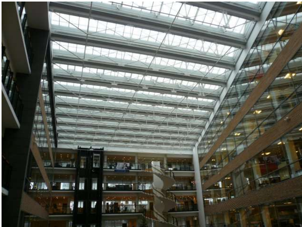
Figure 2.8. The roof of the Atrium.
