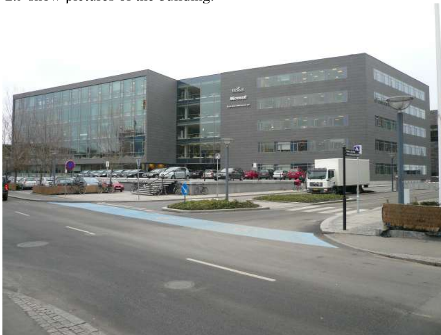
Figure 2.2. The West façade. Orientation: 31° from West towards South.
