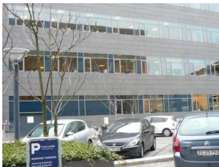
Figure 2.10. Opaque glazing in the façade.
