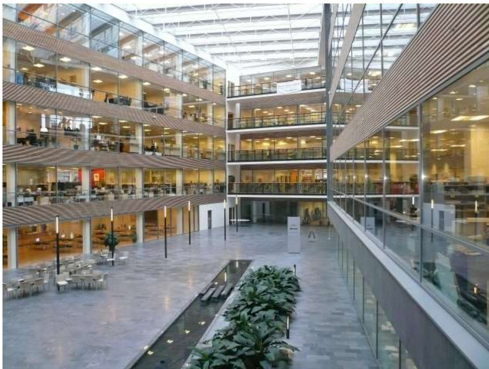
Figure 2.6. The atrium seen towards South.
