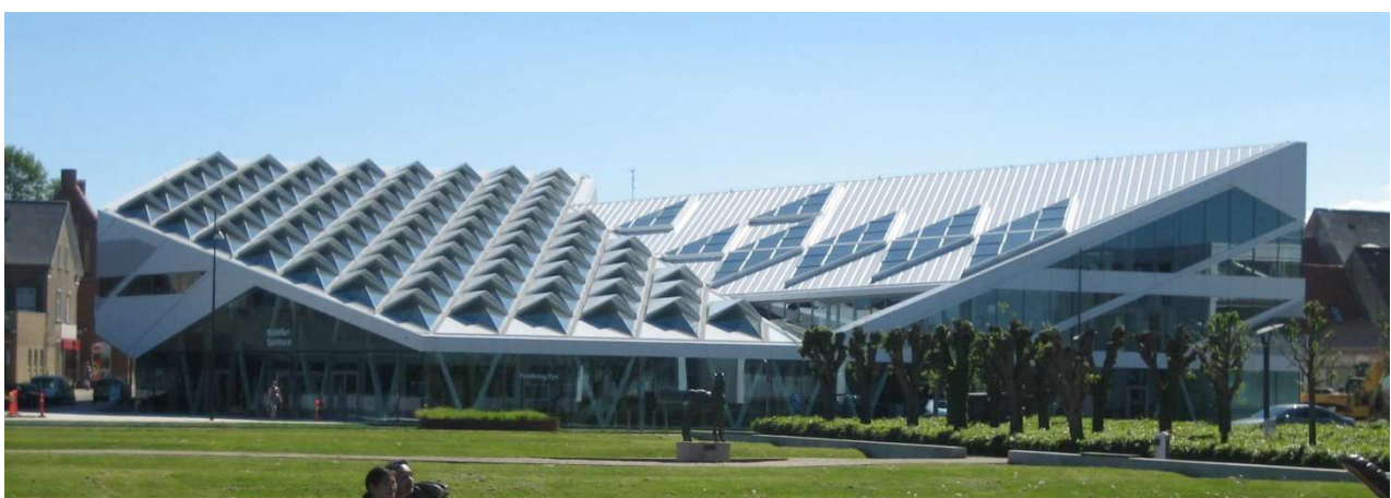
Figure 2. Picture of the North and East façades of the building.
