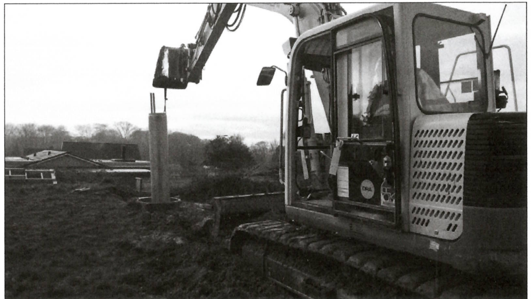
Kappeveksler under montage.
