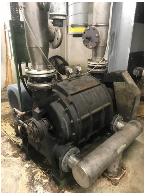
Figur 6.7 Vandringspumpe
